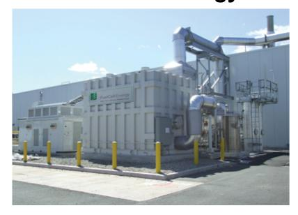
2.8 MW MCFC <50% efficiency ~\$2500/kW
