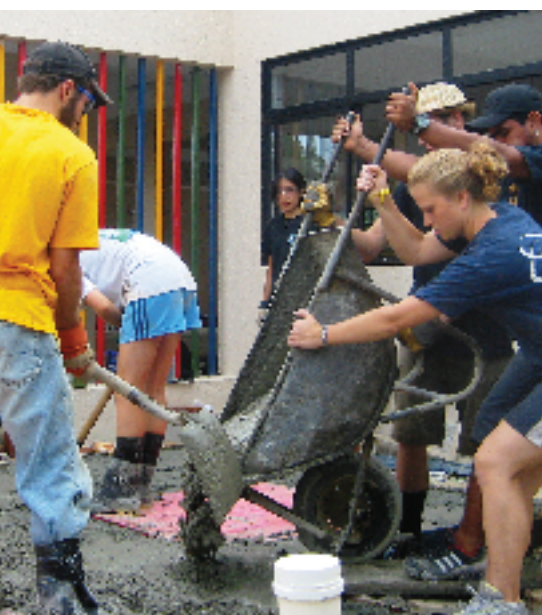
(Left) Elliot Cohen (yellow shirt) works with other EWB students on filling septic tank formwork with concrete in Bebedouro, Brazil. (Above) EWB students Bob Hayes (left, red shirt), and Len Goff (right, red shirt) use their rudimentary French to negotiate for lunch in Dissin, Burkina Faso.
